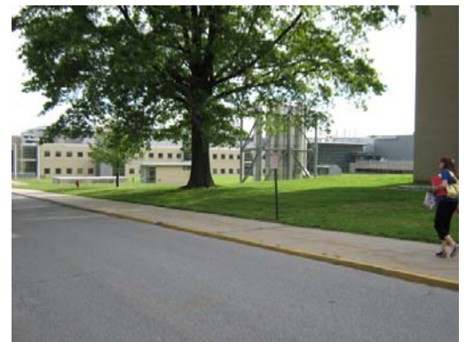
The New N.I.S.T. Gage Calibration Building
